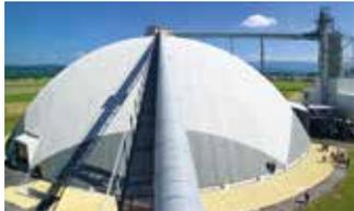
**EFFICIENCY** \_Providing the highest storage capacity per m<sup>2</sup>. Ease of transportation, reduced civil engineering work in large part due to shallower foundations and unnecessary wall enclosures combined with a high precision timber structure enables fast assembly times on client site.
