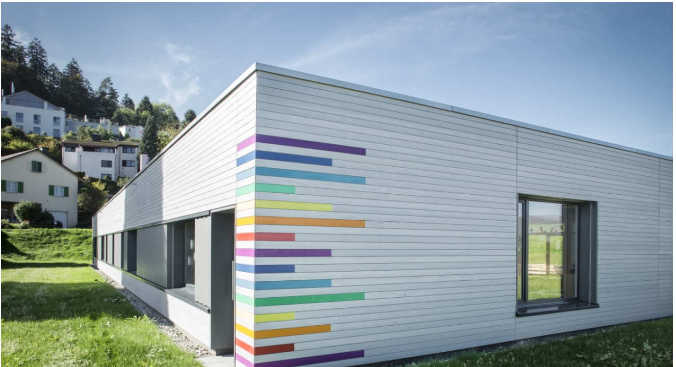
Kindergarten in Killwangen
